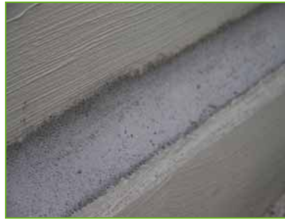
A concave fillet in the wall-floor junction with KOSTER Repair Mortar
