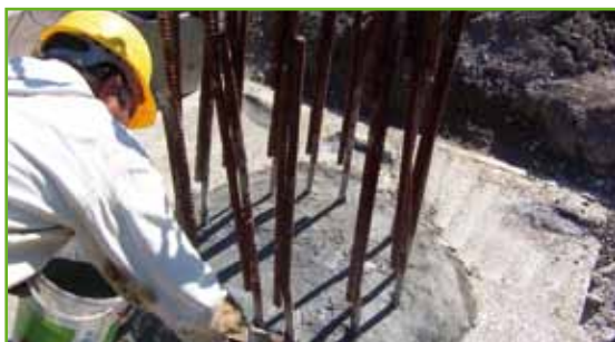
Waterproofing of the pile head with KOSTER NB 1 Grey
