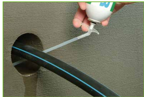
A PU-Foam is injected in order to have a backing for the KOSTER KB-Flex 200.
