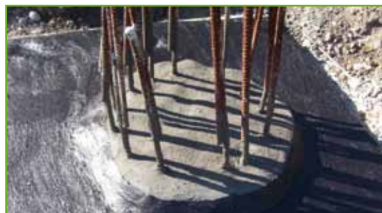
Connection of the area waterproofing (KOSTER Deuxan®) to the pile head waterproofing
