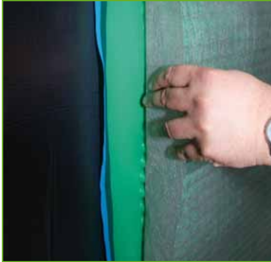
KOSTER SD Sheet 3-400 protects the waterproofing and provides a drainage for residual water.
