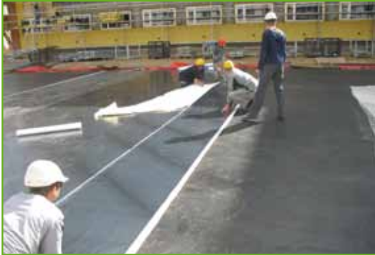
Waterproofing with KOSTER KSK Membranes
