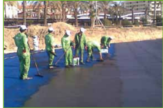
Waterproofing with KOSTER Deuxan®
