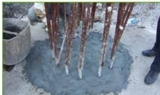
Installing a fillet and smoothing the area with KOSTER Repair Mortar
