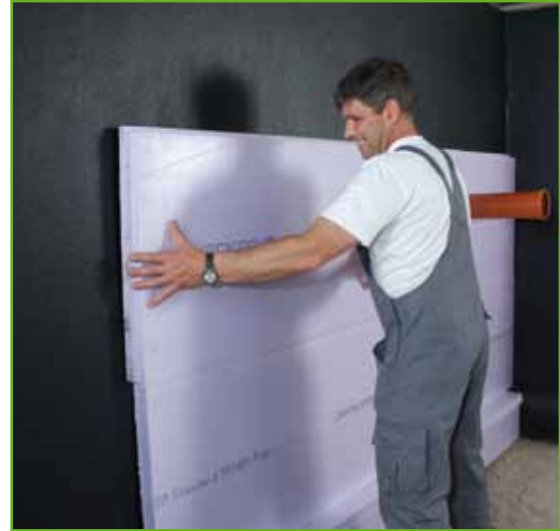
XPS boards bonded with KOSTER Deuxan®
