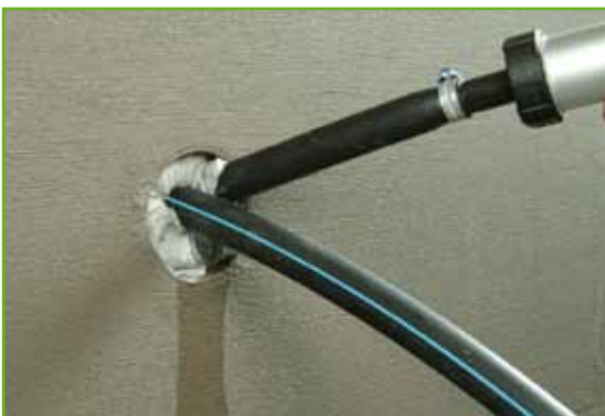
Then KOSTER KB-Flex 200 is filled into the void using the KOSTER Special Caulking Gun.
