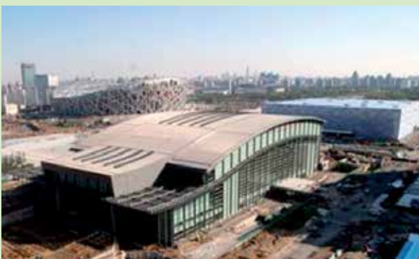
Olympic hall, Beijing, China
