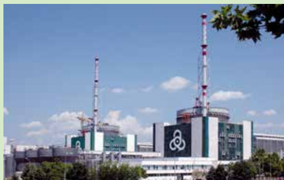
Nuclear power station, Sofia, Bulgaria
