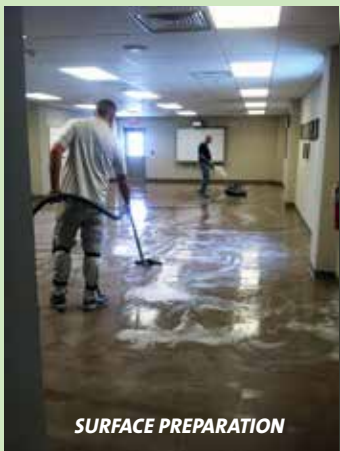
FLOOR READY TO RECEIVE COATING
