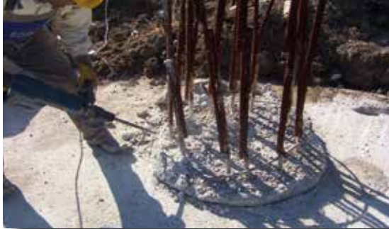
Removing protrusions, cleaning the pile head
