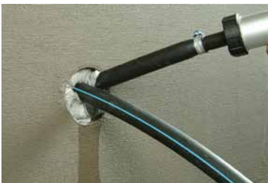
Then KOSTER KB-Flex 200 is filled into the void using the KOSTER Special Caulking Gun.
