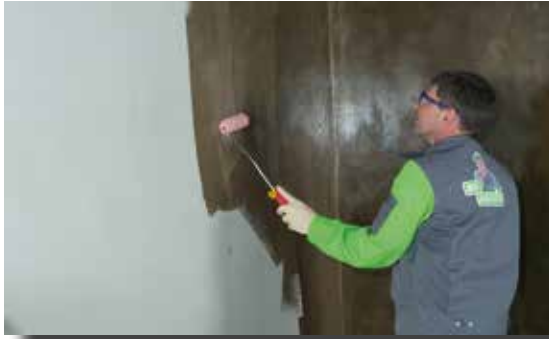
After priming the substrate, fillets are installed in the wall-floor junction.
