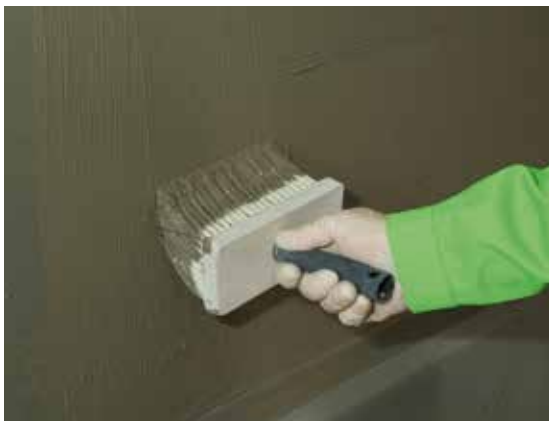
KOSTER NB 1 Grey is applied using a coarse brush.
