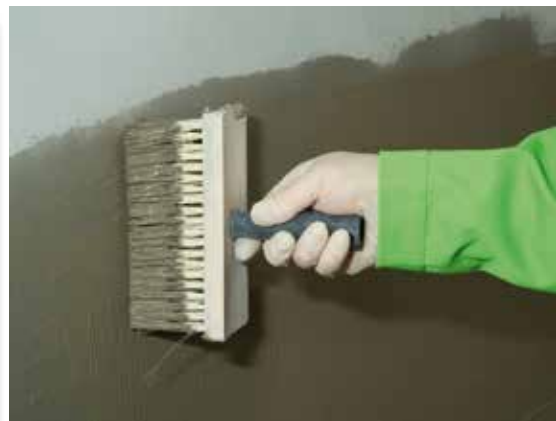
Make sure to brush up and down as well as left and right in order to close all pinholes.
