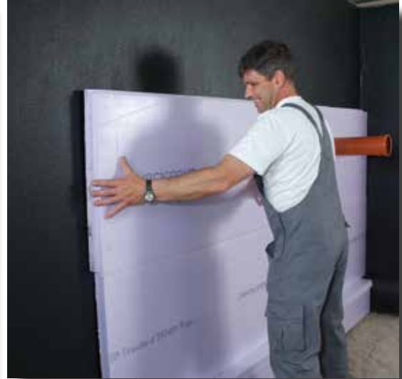
XPS boards bonded with KOSTER Deuxan®
