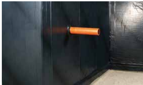
Finished waterproofing with KOSTER KSK.
