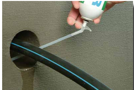
A PU-Foam is injected in order to have a backing for the KOSTER KB-Flex 200.
