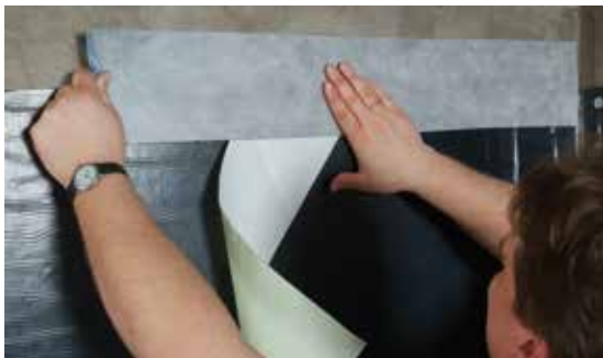
If no separate base waterproofing is installed, the upper edge of the waterproofing layer has to end approx. 12" above grade. In order to achieve an attractive visual appearance, the upper edge of the membrane can be covered with the cold self-adhesive KOSTER Butyl Fix-Tape Fleece. This tape can be plastered over.
