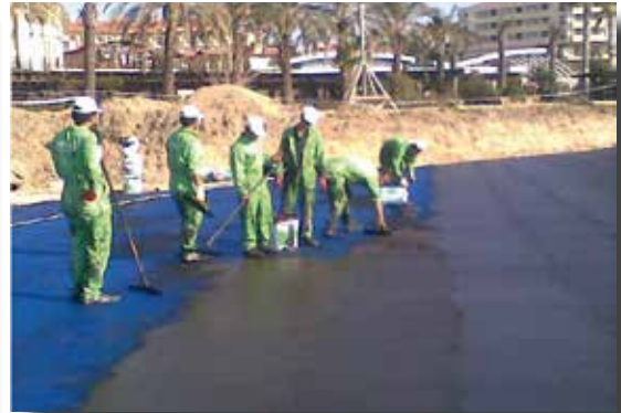
Waterproofing with KOSTER Deuxan®
