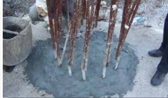
Installing a fillet and smoothing the area with KOSTER Repair Mortar
