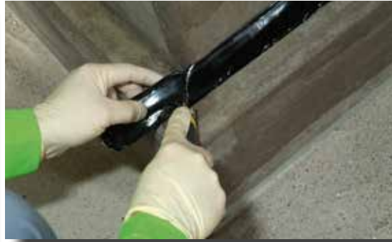
Fillets can be made of either KOSTER Repair Mortar or alternatively using the cold self-adhesive KOSTER KSK Triangular Ribbon.
