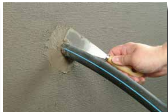
The pipe penetration is now waterproof. In order to protect the waterproofing the area around the pipe or cable is plugged with KOSTER KB-Fix 5.
