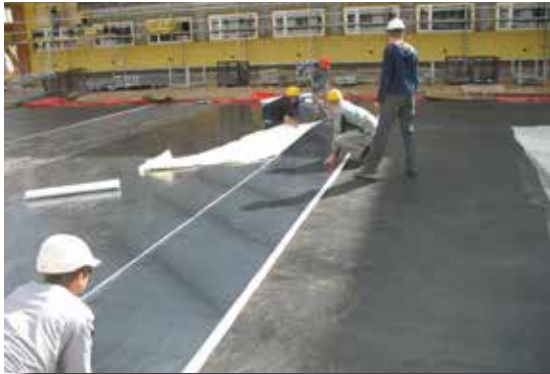
Waterproofing with KOSTER KSK Membranes
