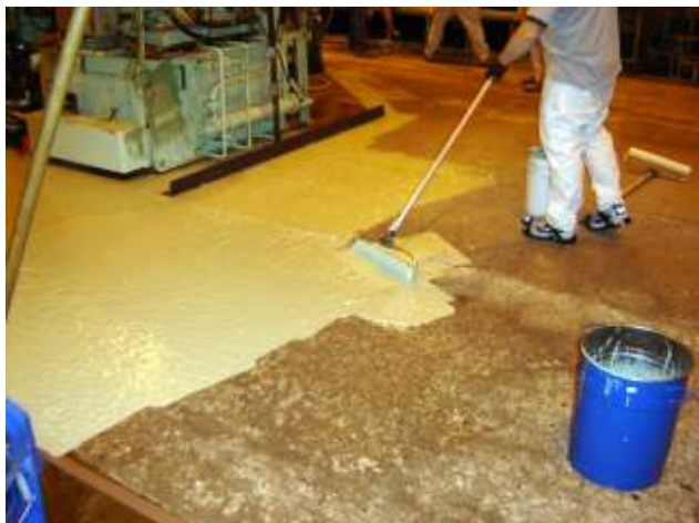
Squeegee operations over the rough substrate. This proved to be difficult as the material tended to "pond" in the low areas, pits and holes.
