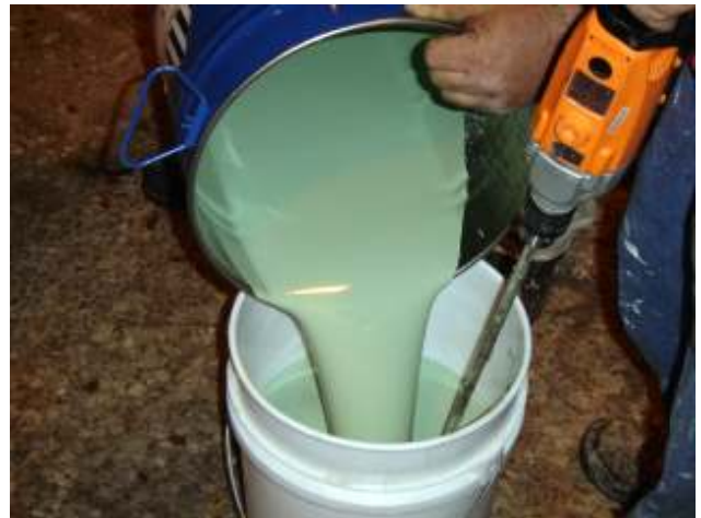
After mixing the ORS-C for approximately 3 minutes, it is poured into another bucket for distribution on the floor.
