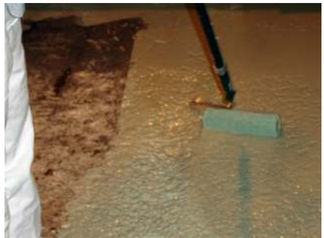
In this application a 9" roller was the best for application of the ORS-C. This allowed the material to be applied evenly with little ponding.
