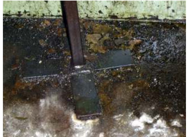
This area is directly adjacent to the previous photo and also shows extensive oil and grease build-up. The concrete appears to be uncoated in these areas.
