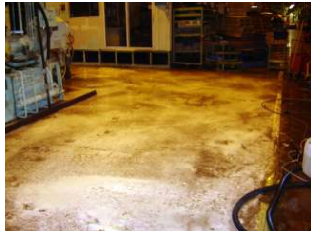
Second application of foam down and a 50 minute or so wait follows. When the foam turns clear it is a good indication of the proper time.
