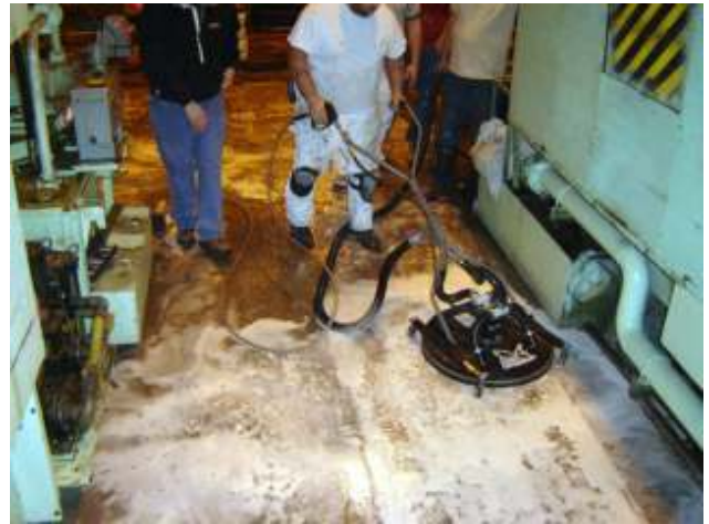
Junior takes over spinner operations. This high pressure procedure forces the detergent into the concrete for deep cleaning action.
