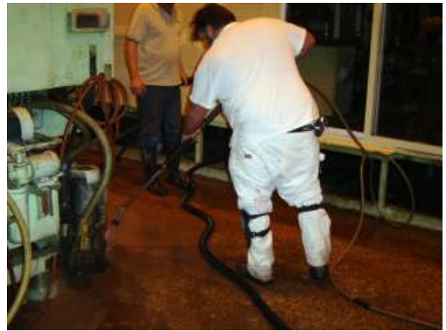
Rinsing continues with Joachim standing by with a vacuum to remove and control water flow.
