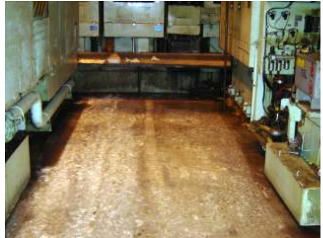
The left leg of the "U". Cothern Bros. has already pre-profiled the surface to an approximate CSP 5-6. Note the dark areas at the edge of the machinery, oil.
