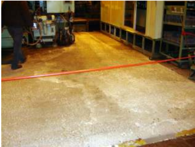
Floor area to be coated with the ORS treatment. This is the right leg of the "U" shaped area. This area has been subjected to oil contamination.
