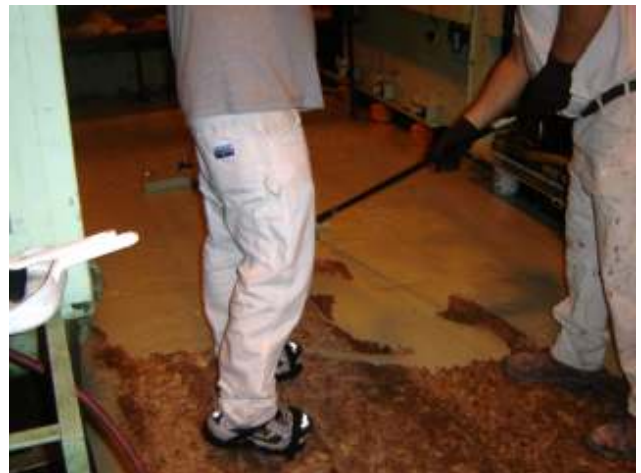
After cutting in, rolling operations started. The crew started coating using a squeegee and an 18" roller.
