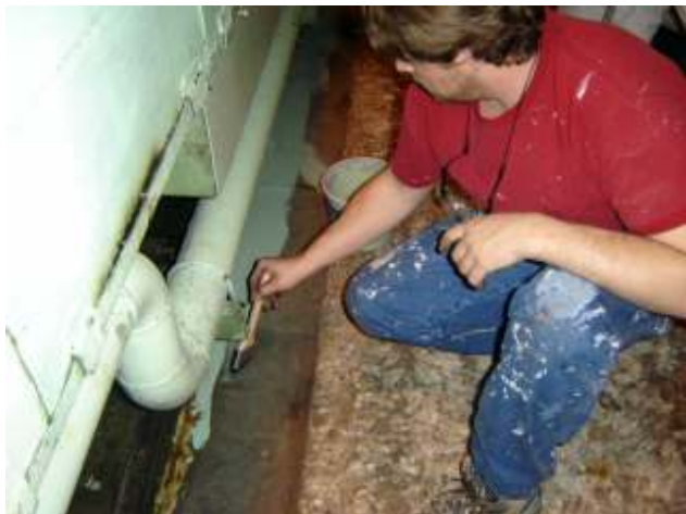
Here Tom is cutting in around the perimeter of the area. You must be careful not to get this application too thin, the proper millage rate must be maintained.
