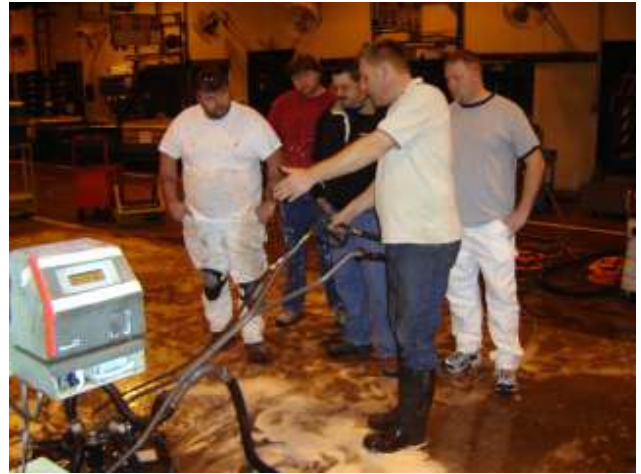
Joachim gives the crew instructions on how to proceed with the high pressure floor spinner to deep clean the substrate.
