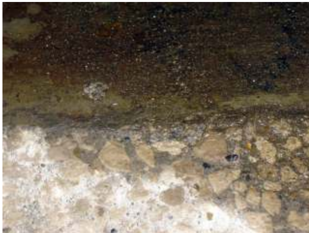
This photo shows clearly the demarcation line between the oily substrate and the machined surface profiled area with aggregate showing.
