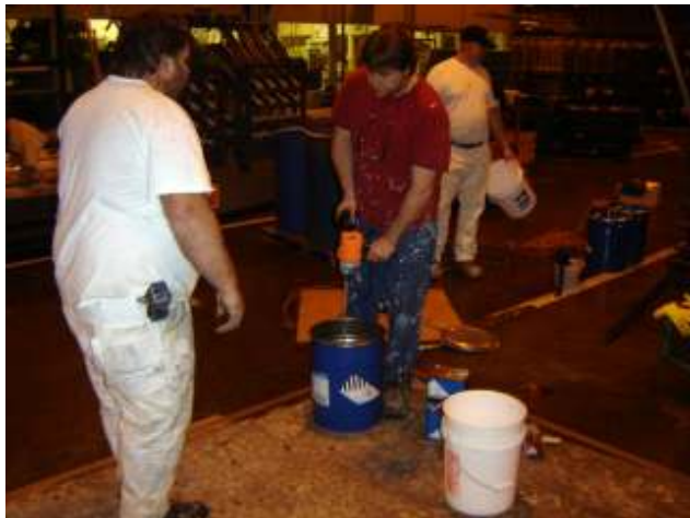
Tom starts mixing procedures with the ORS-C primer coating. Tom is using a 1/2" drill and a jiffy mixer.
