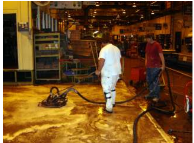
Wrapping up the spinning operation. At this point Junior is letting the vacuum action remove some of the excess water on the deck.
