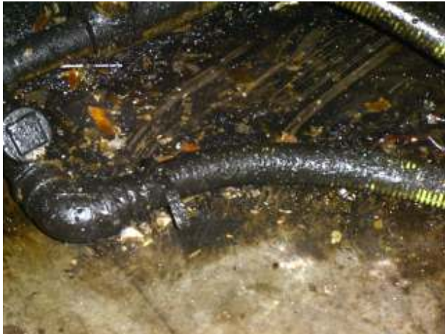
A close up of the oil and grease build up near the machine. You can see the edge of the floor preparation near the hose.
