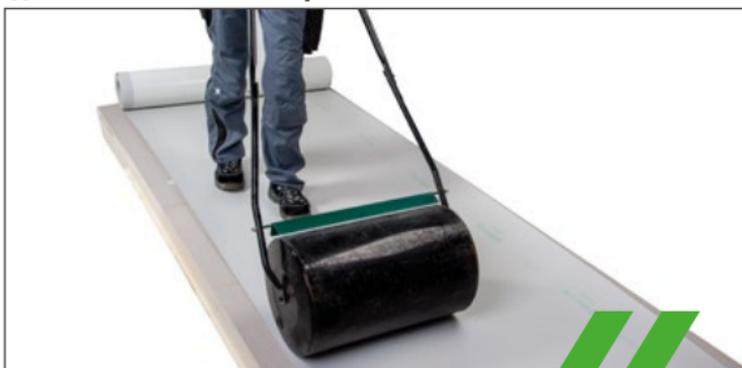
// The Membrane is then be pressed on over the entire surface, ideally with a pressure roller.
