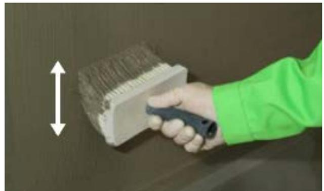
After the material has cured, the KÖSTER Restoration Plaster Key is splashed onto the substrate so that the plaster key is no thicker than 5 mm and covers approximately 50 % of the area. This step will ensure the optimal adhesion of the KÖSTER Restoration Plaster.
