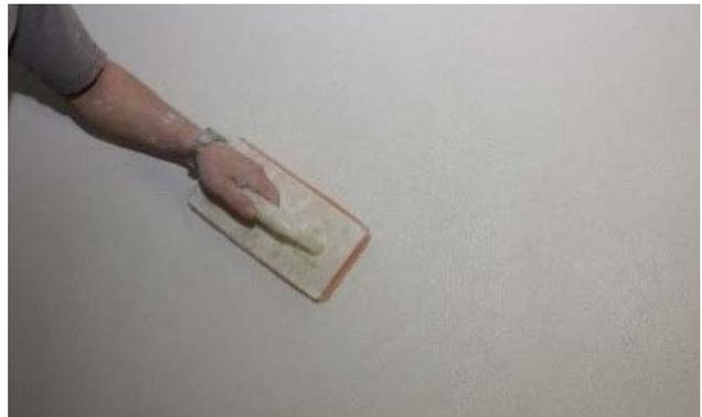
KÖSTER Restoration Plaster allows the masonry to dry without damage. KÖSTER Restoration plaster is hydrophobic and open to vapor diffusion. Salts remaining in the wall are absorbed by the KÖSTER Restoration Plaster preventing salt efflorescence and damage to the plaster or paint. Various KÖSTER Restoration Plasters are available (Grey, White, Fast and Light). KÖSTER Restoration Plaster
