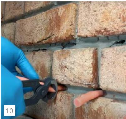
10 After applying the injection, the capillary rods remain in the masonry. Protruding ends are pulled out and cut off.
